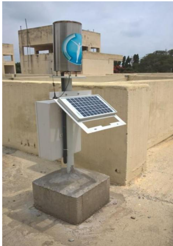
Figure 1: Installed Rainwater Sensor
